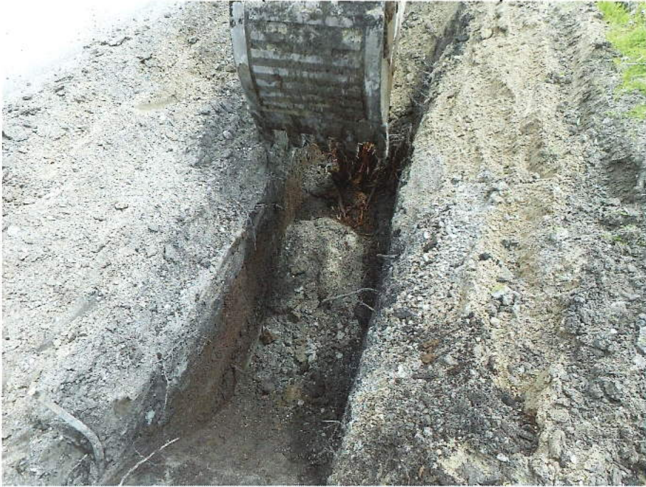
TRENCH INVESTIGATIONS – CRUSHED STONE. NO FILTER PHOTO SET 2 (BEFORE STONE ADDED)
