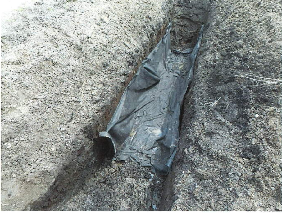
TRENCH INVESTIGATIONS – CRUSHED STONE. FILTER FABRIC PHOTO SET 3
