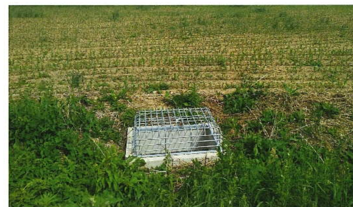
PHOTO OF TYPICAL BIRDCAGE GRATE REQUIRED ON 900x1200mm CATCHBASIN
